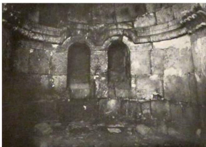
Al-Ruṣāfa: Alamundarus church_above longitudinal_interior of the main apse
