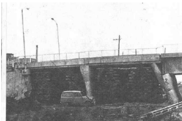
a) Damage of the abutment and piers in the Yachiyo Bridge, 1964 Niigata Earthquake (Abdoun and Dobry 2002).
