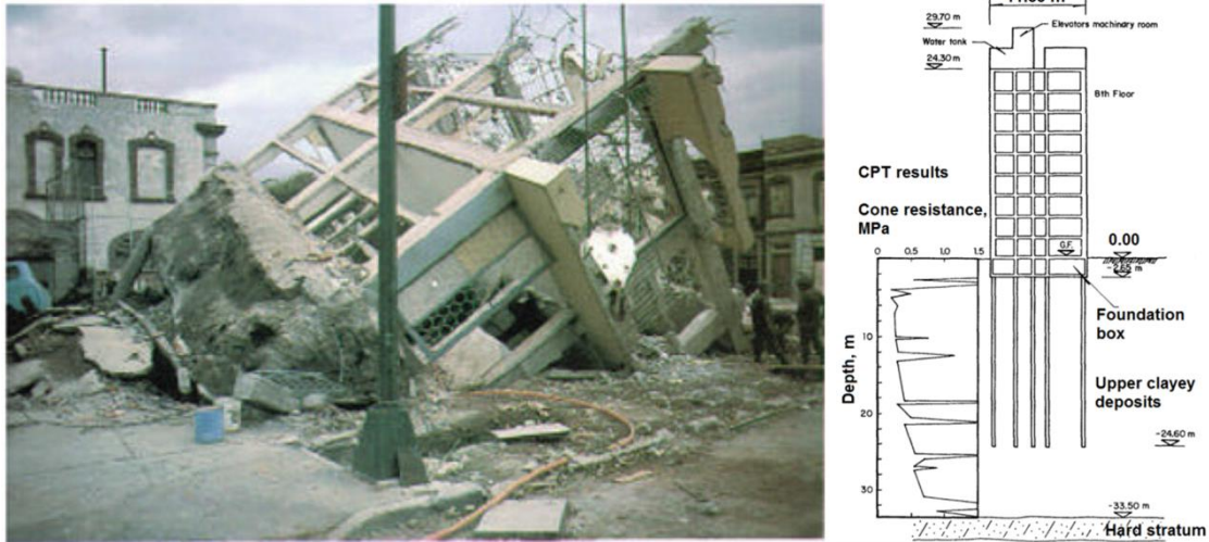
a) Building collapse during the 1985 Mexico City Earthquake. Foundation and geotechnical conditions (Mendoza and Auvinet 1988).
