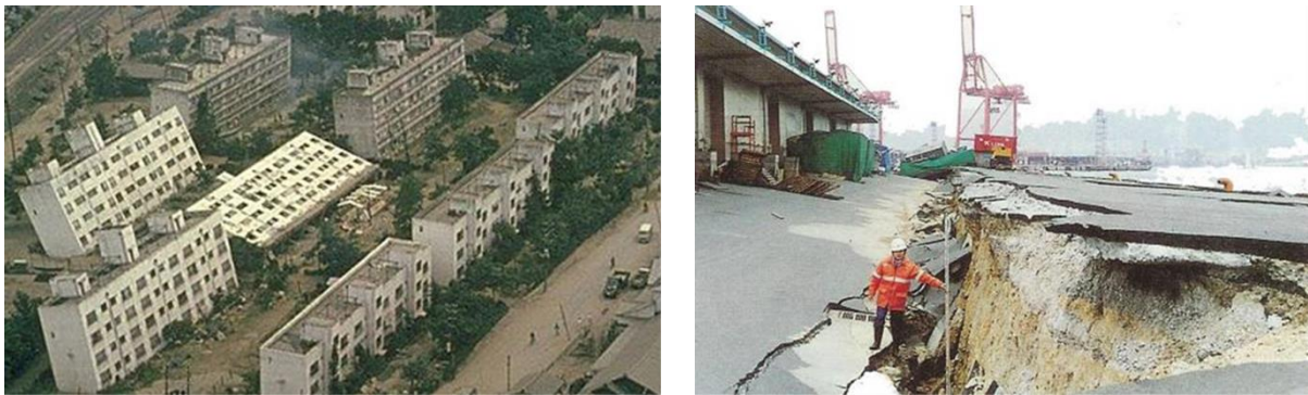
a) Building toppling Niigata 1964
