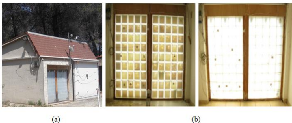
Figure 3-2: (a) TIM-PCM wall from the outside, (b) PCM in solid phase (left) and liquid phase (right), from the inside
