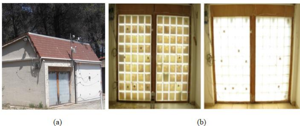
Figure 1-9: (a) TIM-PCM wall from the outside, (b) PCM in solid phase (left) and liquid phase (right), from the inside (PERSEE center in Sophia Antipolis)
