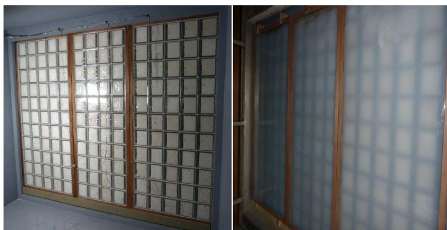
Figure 1-10: Interior and exterior photo of the TIM-PCM wall of CETHIL
