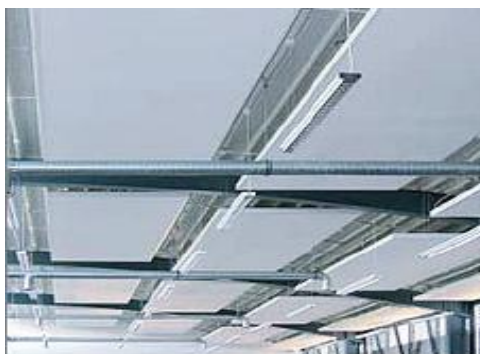
Figure 0-44: Installation of ILKATHERM PCM board [108]
