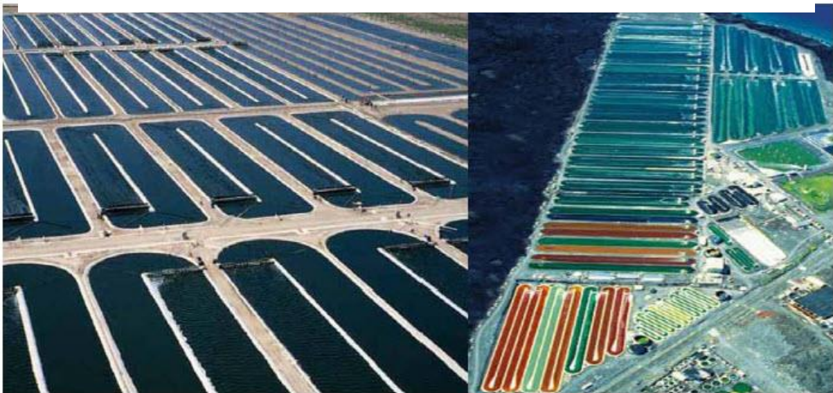
Figure 40: Open raceway ponds for commercial microalgae production (Source: Global CCS Institute). Left image: Spirulina production, Ponds ~ 1 acre (Earthrise Nutritionals, LLC, California); Right image: Haematococcus pluvialis (red ponds) and Spirulina (Cyanotech Co., Hawaii).
