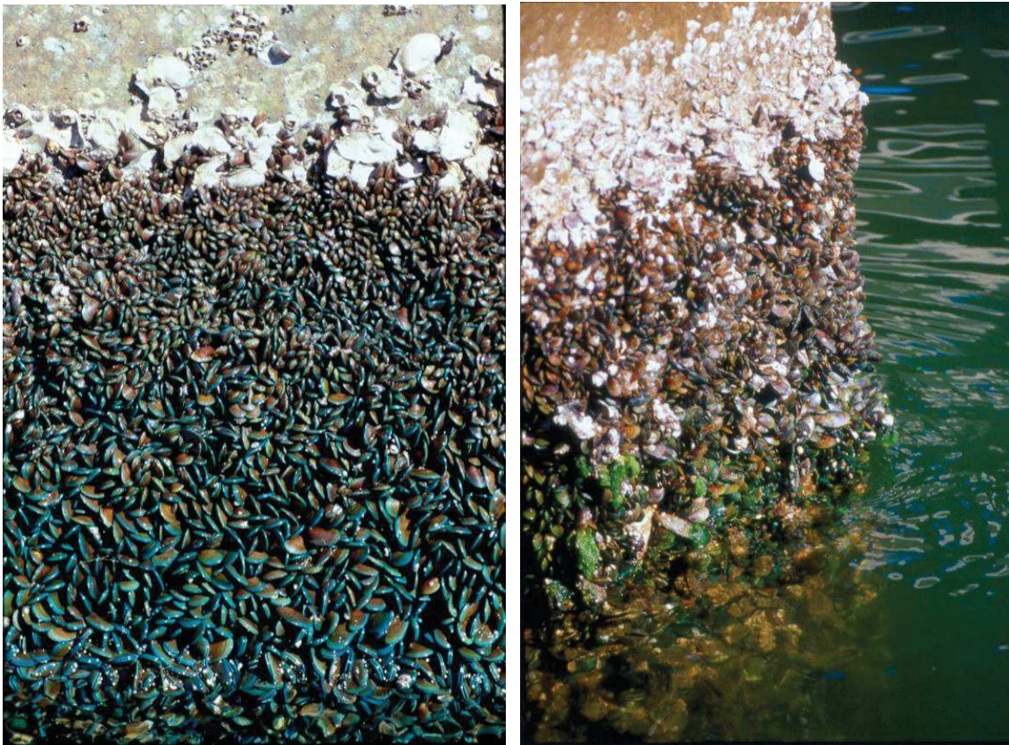
Figure 3: Dense settlement of green mussels on top of oysters on Gandy Bridge, Tampa Bay Florida (Photos by Dr. Patrick Baker, University of Florida)
