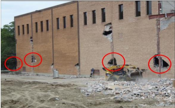
Figure 2. 4 The circled columns on North Side of the Building were Removed During the Experiment (Sezen and Song, 2009)
