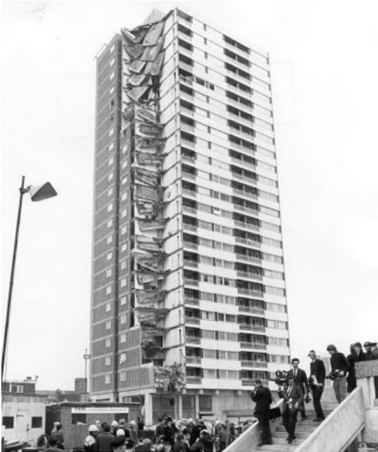
Figure 1. 1 Ronan point apartment collapse, 1968
