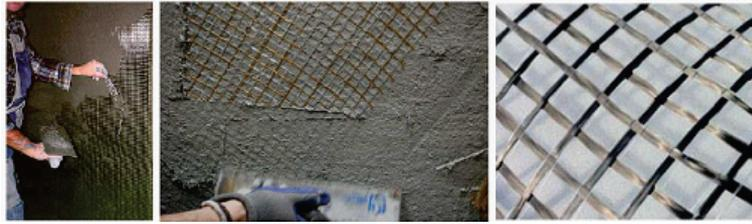
Figure 1.1: FRCM Fibre Reinforced Cementitious Matrix.
