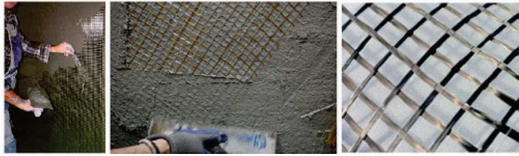
Figure 1.1: FRCM Fibre Reinforced Cementitious Matrix.
