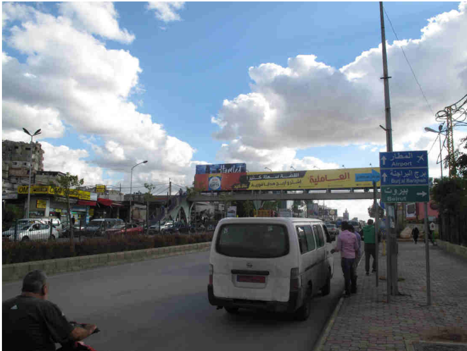
Figure 5-23: Pedestrian bridge at the entrance of Bourj el-Barajneh Camp
