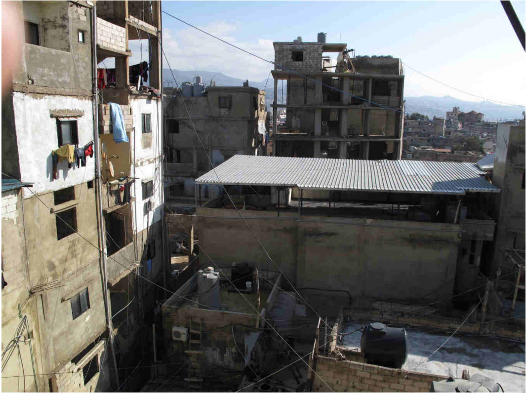
Figure 7-9: Vertical growth Five new stories between 2012 and 2018 in the building to the left, and three new stories in the building in the center. February 2018
