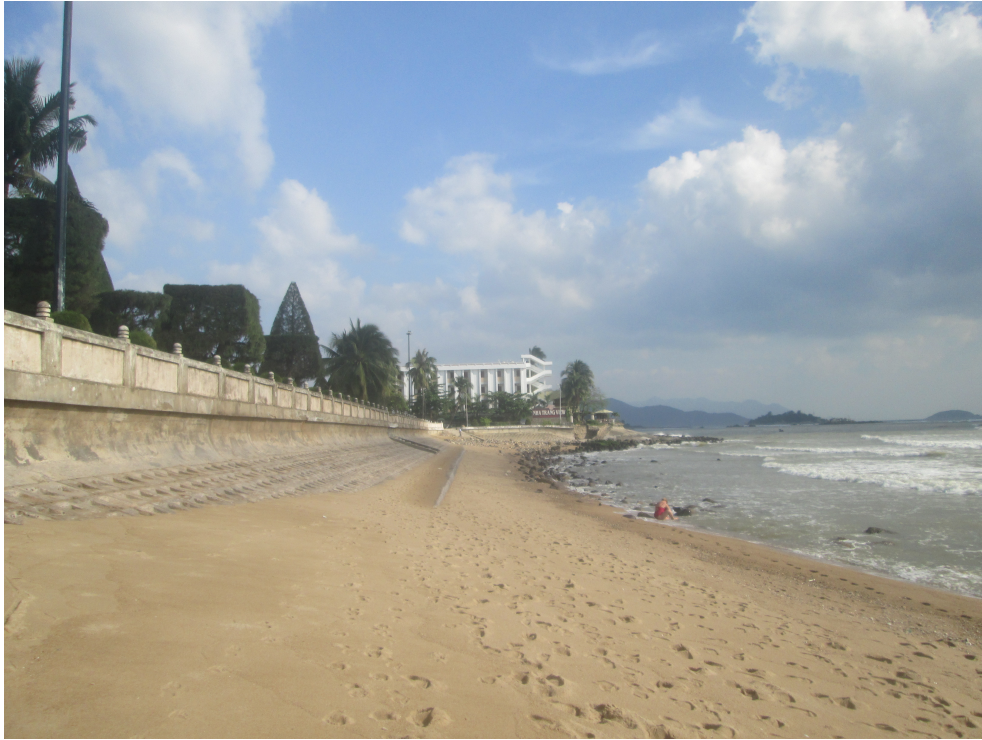
Figure 2.14: A part of the vertical and sloping seawall along the stretch between Nha Trang View restaurant and the structure Hoa Bien.
