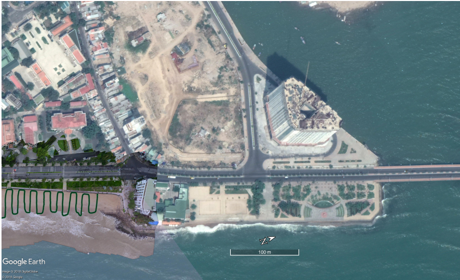
Figure 2.10: Concrete constructions around the northern section of Yersin Park at the river mouth of Cai river. From Google Earth Pro.
