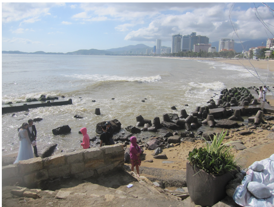
Figure 2.13: Two jetties made from tetrapods at the south of Nha Trang View restaurant. Photo taken at 09h22 06/12/2015.
