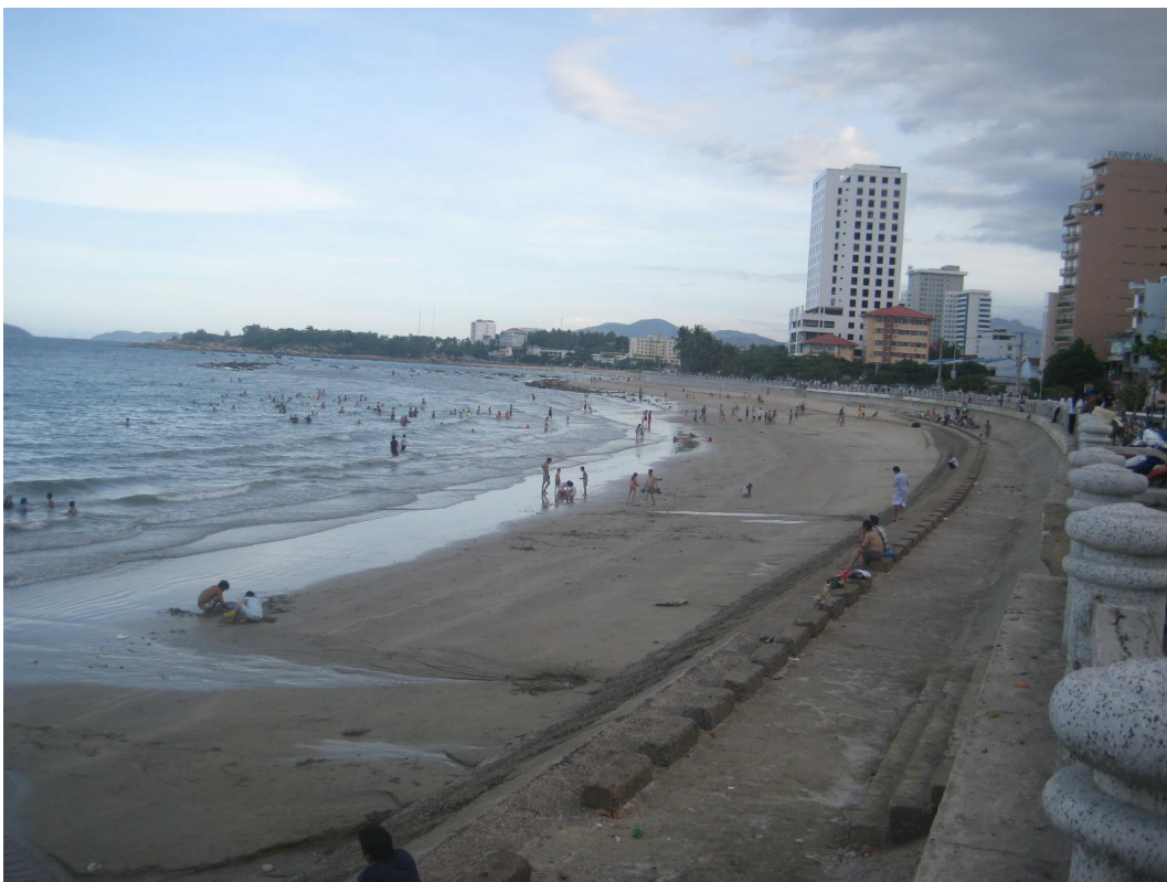
Figure 2.5: The beach of Cai river mouth has suffered from severe erosion and today the beach is absent and only the seawall is visible. Photo taken at 16h51 24/05/2013.
