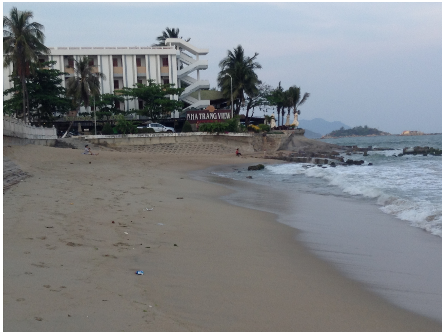
Figure 2.12: The seawall and the groins at the beach south of Nha Trang View restaurant. Photo taken at 11h14 12/03/2015.
