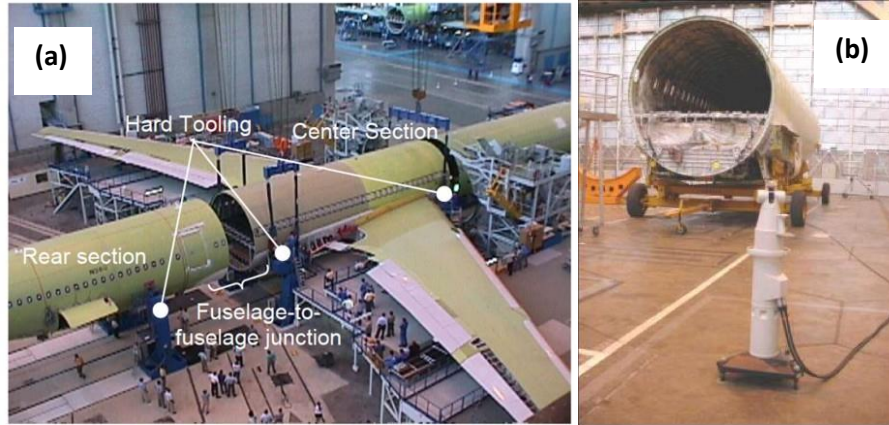
Fig. 1.3. Aeroplane assembly. (a). Traditional assembly based on hard tooling. (b). Measurement-assisted assembly using laser trackers.
