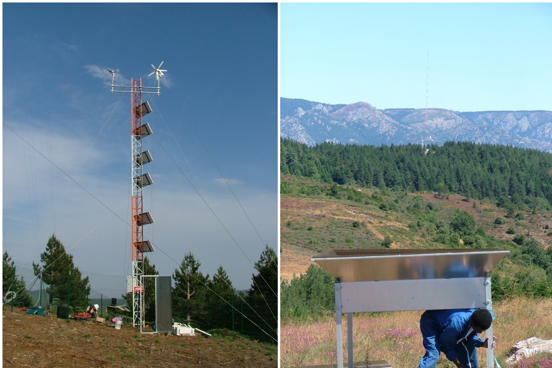
(a) Meteorological mast equipped with anemometers and wind vanes. (b) Sound Detection And Ranging (SODAR) in hilly terrain.
