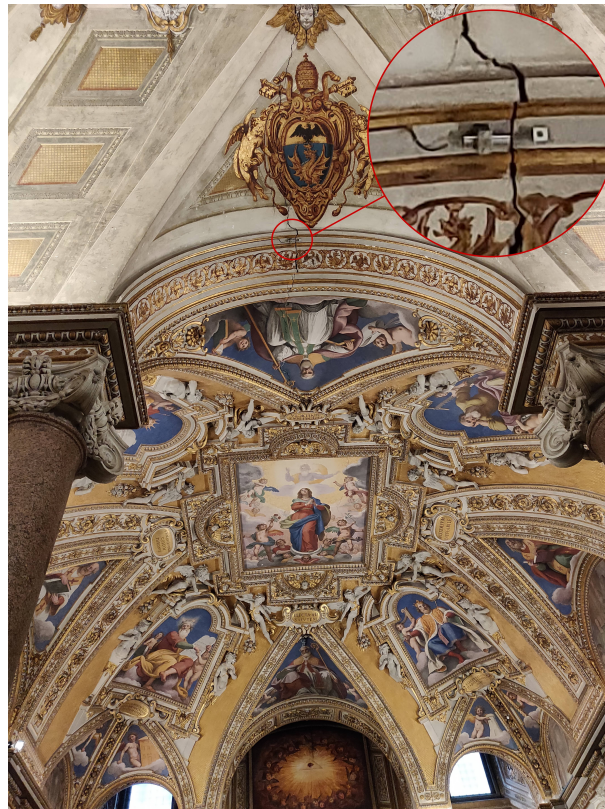
Figure 2: Monitoring of crack opening at Basilica Papale di Santa Maria Maggiore (Photo credit: T. Heitz)
