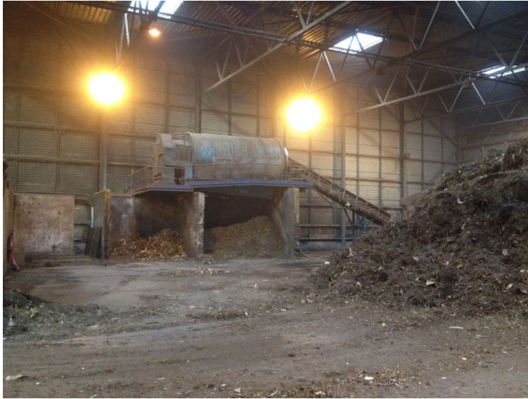
Figure 37 : Installation de compostage de Saint-Ouen-l'Aumône, hall A.
