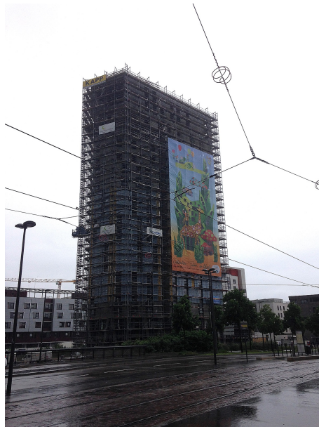
FIGURE 2.1 – La Tour Elithis Danube en construction, mai 2017
