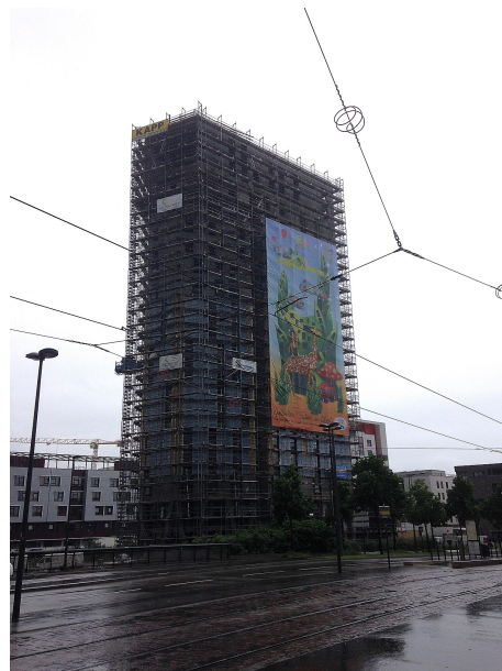
FIGURE 2.1 – La Tour Elithis Danube en construction, mai 2017
