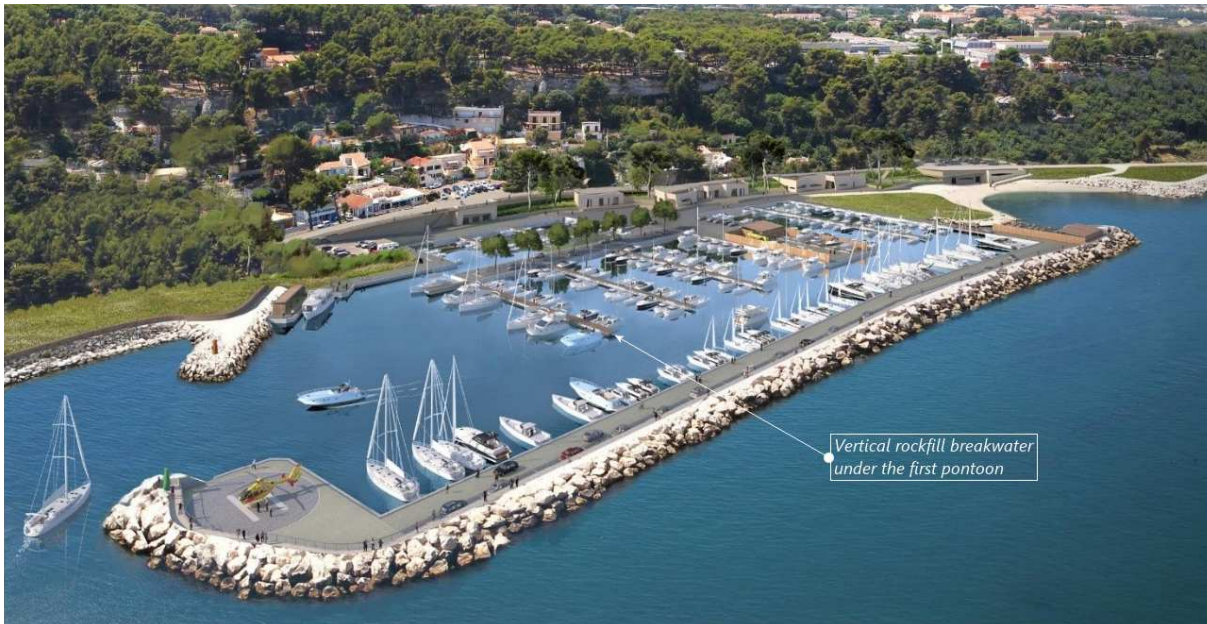
Figure 4.1: 3D view of Istres harbour with the spot of the interested pontoon
