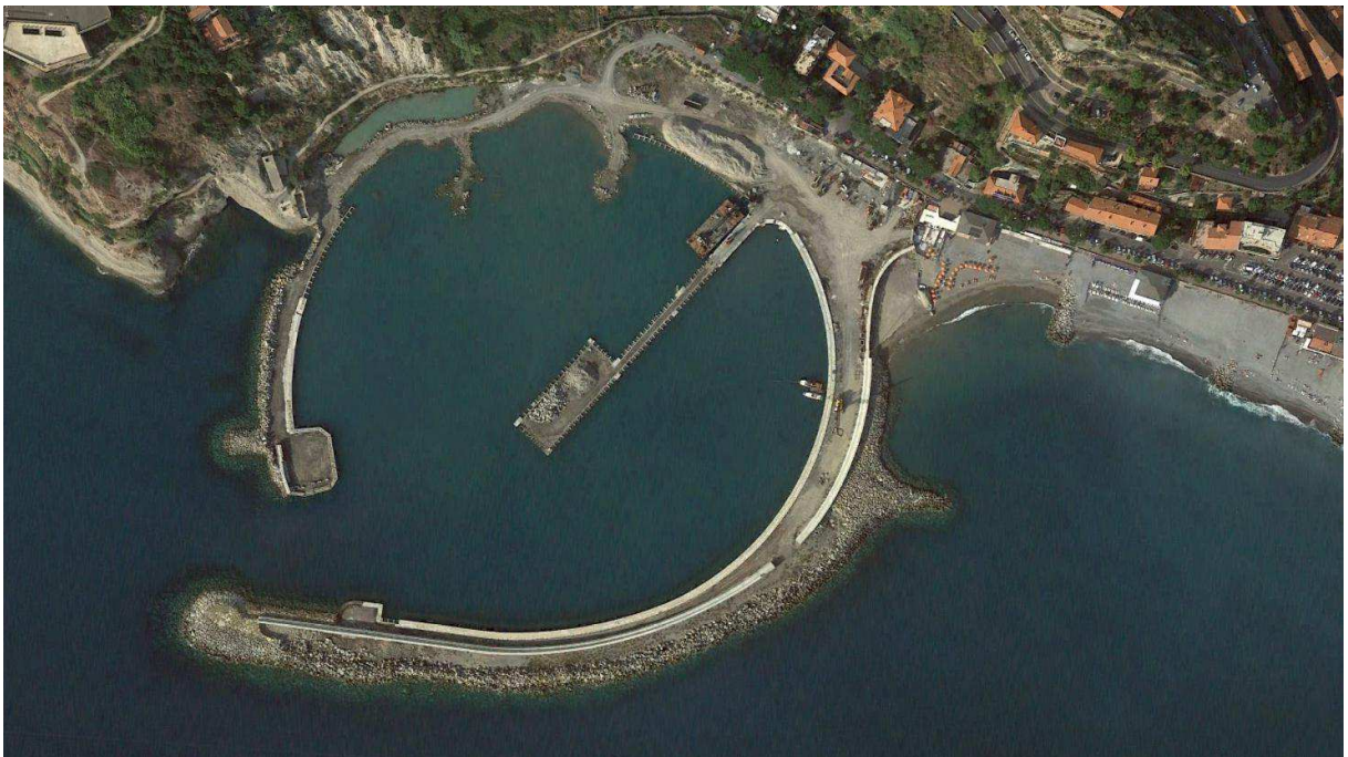
Figure 3.1: State of the port before further constructions, Vintimille
