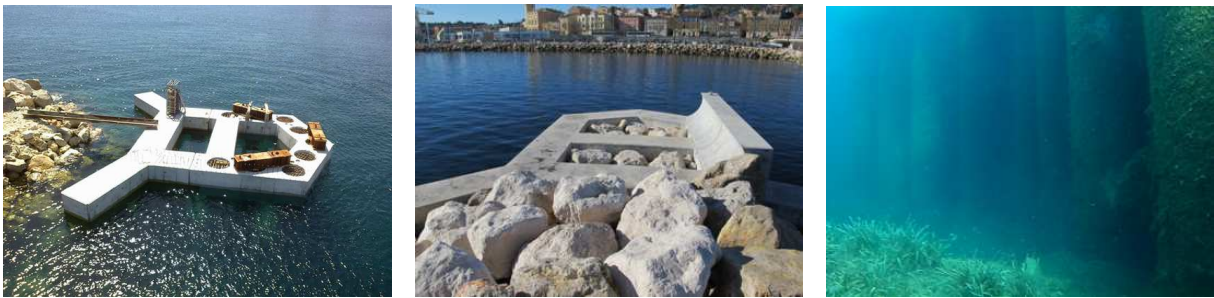
Figure 4: Vertical riprap breakwater in the entry of the port of La Ciotat.
