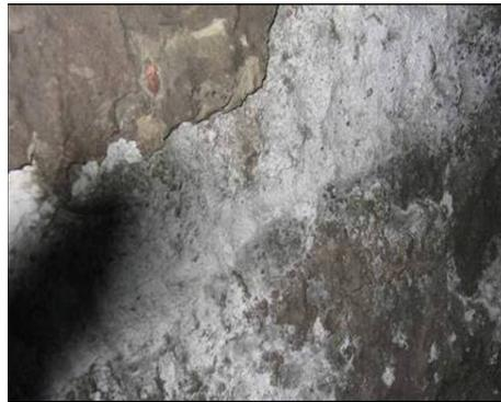
Figure 1.2 – Surface concrete spalling exposed to sulfate-rich environment [4].
