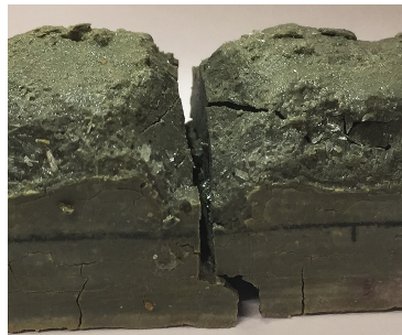
Figure 3.2 – Crystals observation in the cracks of Coupling specimens.
