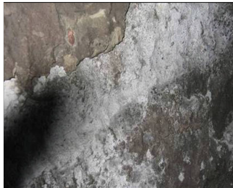
Figure 1.2 – Surface concrete spalling exposed to sulfate-rich environment [4].
