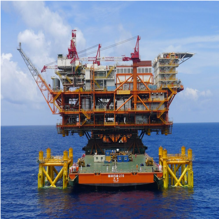
Figure 5 – Floatover installation of a topside 9
