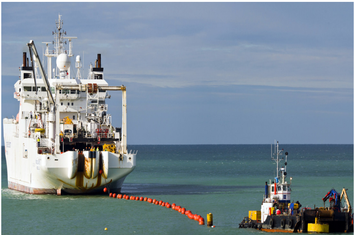
Figure 7 – Power cable laying 11 . The buoys indicate the cable position.
