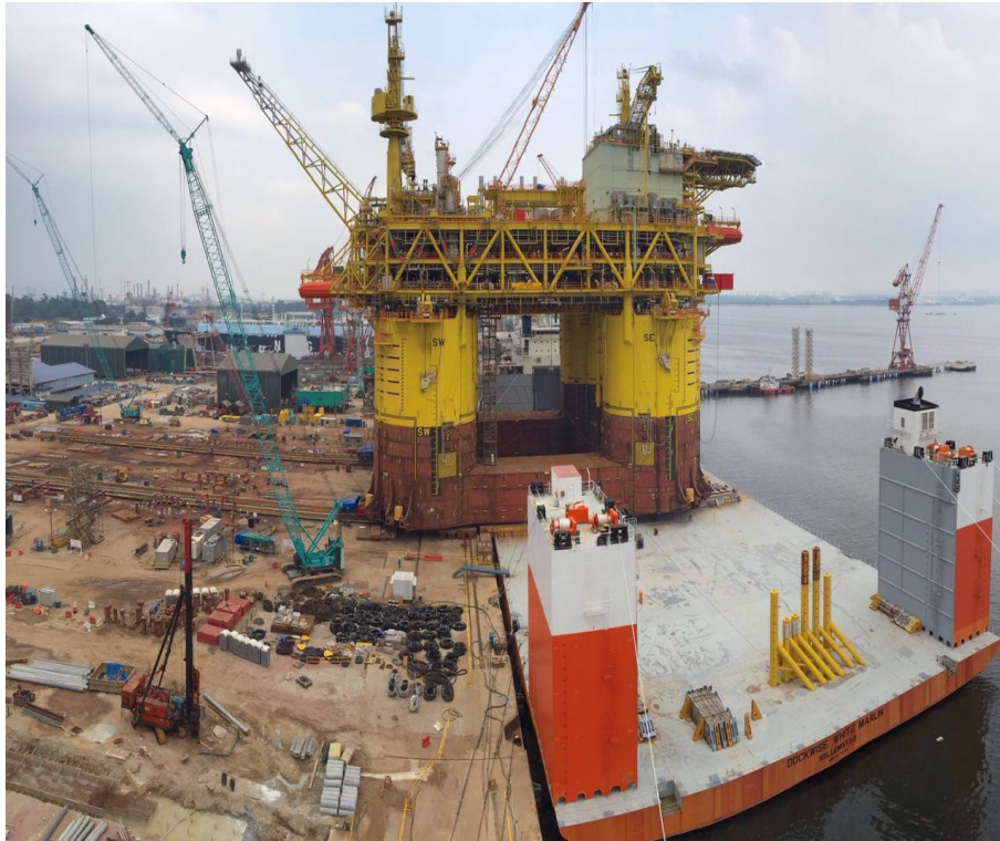
Figure 6 – Loadout of a tension-leg platform using skid rails 10
