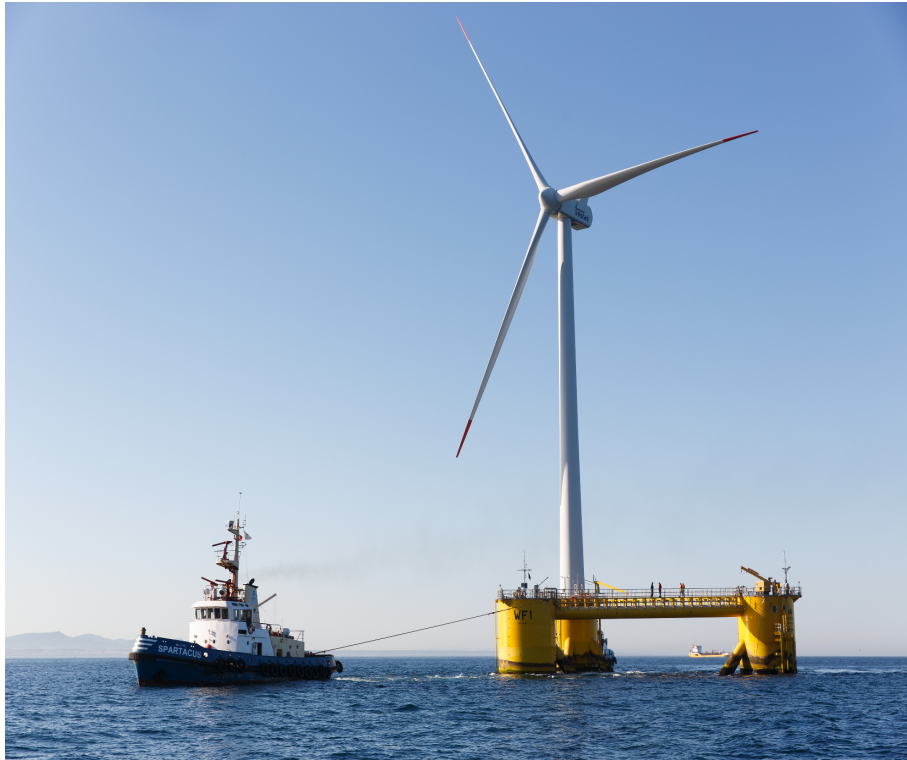
Figure 2 – Towing of the floating wind turbine WindFloat 6
