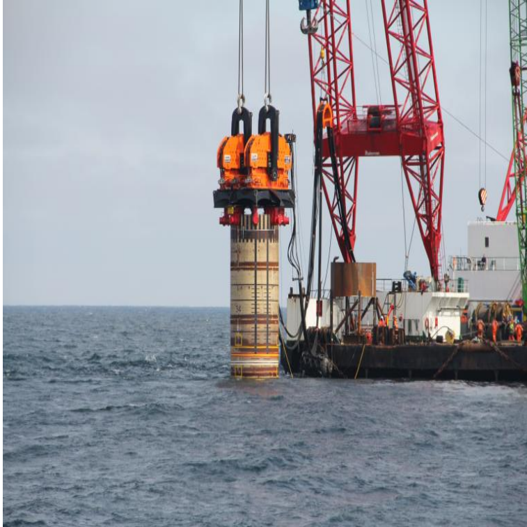
Figure 8 – Piling operation of a monopile 12
