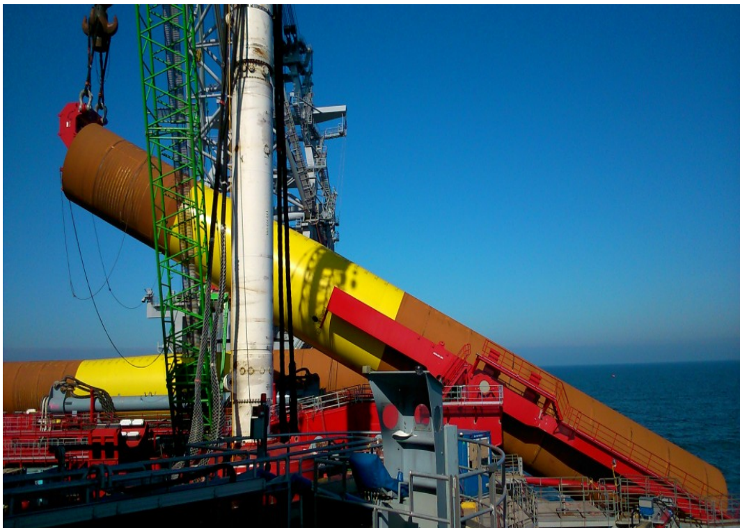
Figure 3 – Upending of a monopile 7
