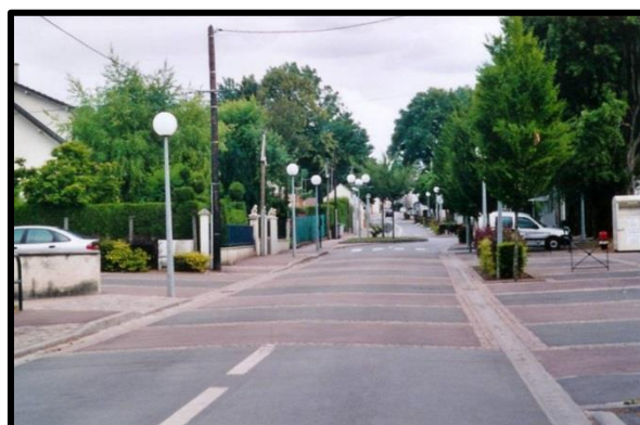
Figure 5.14: Bandes d'alertes transversales (Survilliers, France)
