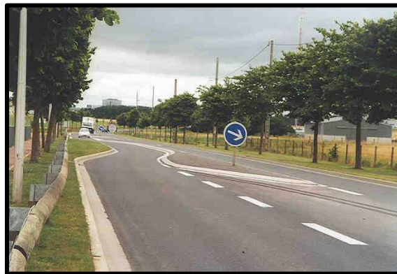
Figure 5.6 : Chicane (D226, Cuverville, France)
