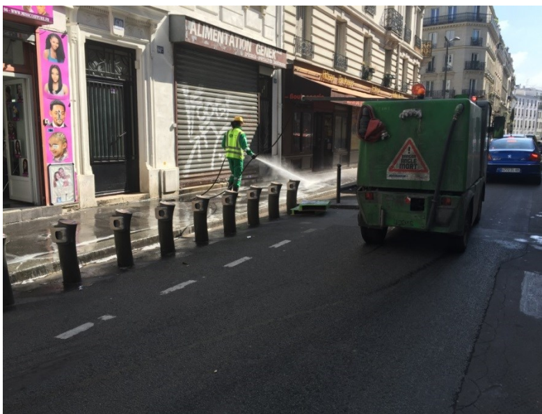
Fig. 2.5 Practice of street cleaning in Paris leading to sediment entering into the combined sewers (photo by G. Shahsavari).
