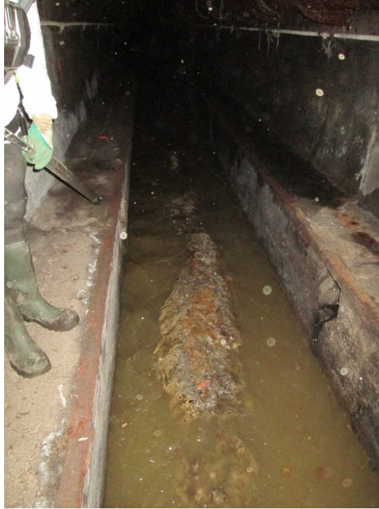
Fig. 6.15 Example of the accumulated rags in the studied channel.
