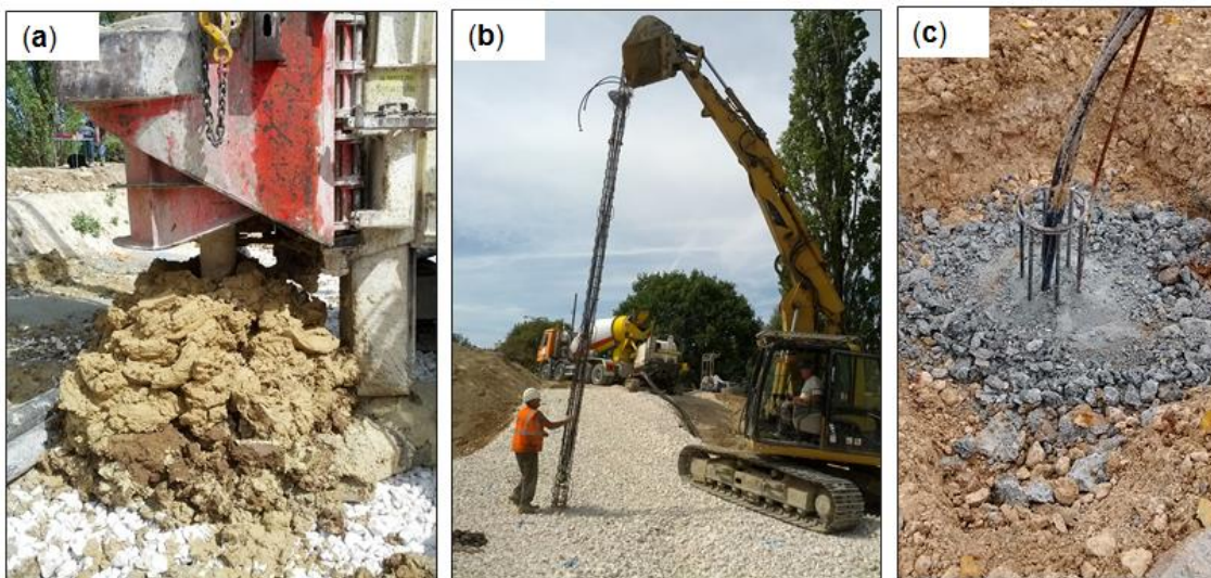
Figure 2-22 Pile installation by continuous flight auger (CFA) method: (a) Drilling, (b) The reinforcement cage is being prepared before being lowered in the fresh concrete column (c) The pile head after teaming.
