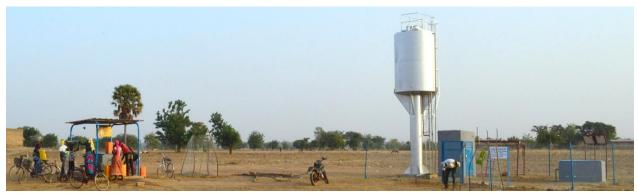
Figure II-9 – Overview of the PVWPS. On the left: the fountain where the inhabitants collect water. On the right: the PV array and the water tank surrounded by a wire netting.
