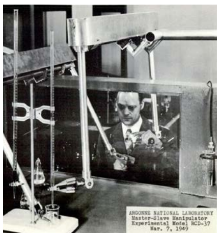
(a) The first master-slave mechanical system.
