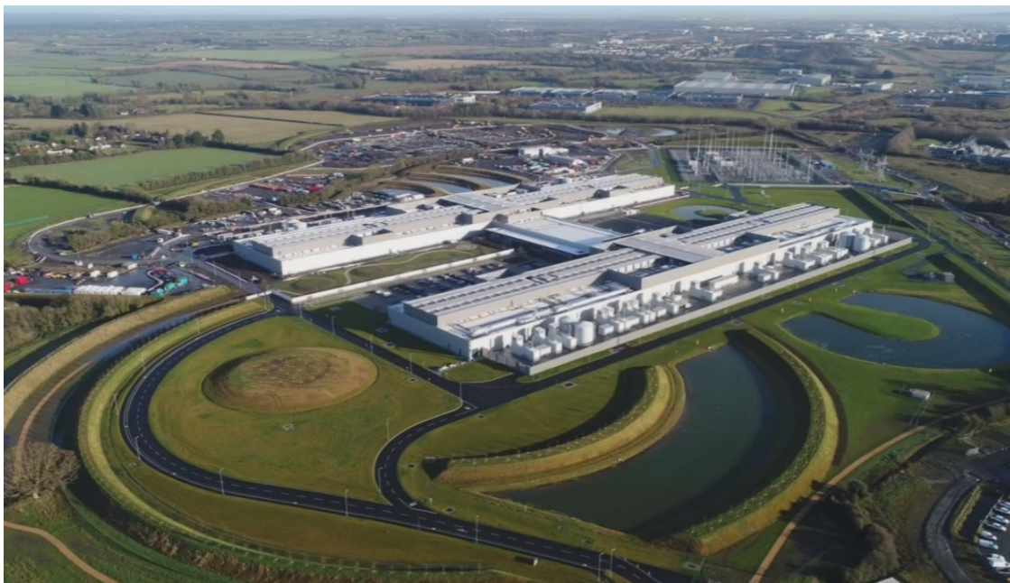
Figure 3.2: Aerial view of the Facebook DC [53]
