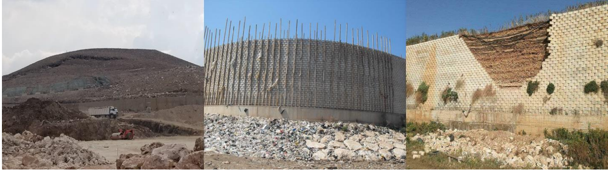
Figure 12: Tripoli's coastal landfill with its protective peripheral wall
