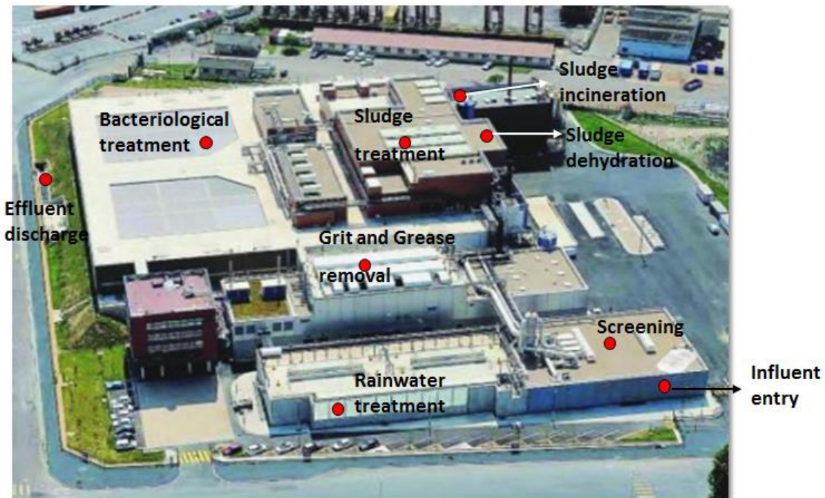
Figure 14: Aerial view of Edelweiss WWTP with its various treatment steps (adapted from the report of CODAH, 2013).
