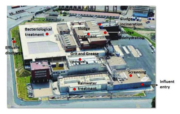
*Figure 14:* Aerial view of Edelweiss WWTP with its various treatment steps (adapted from the report of CODAH, 2013).
