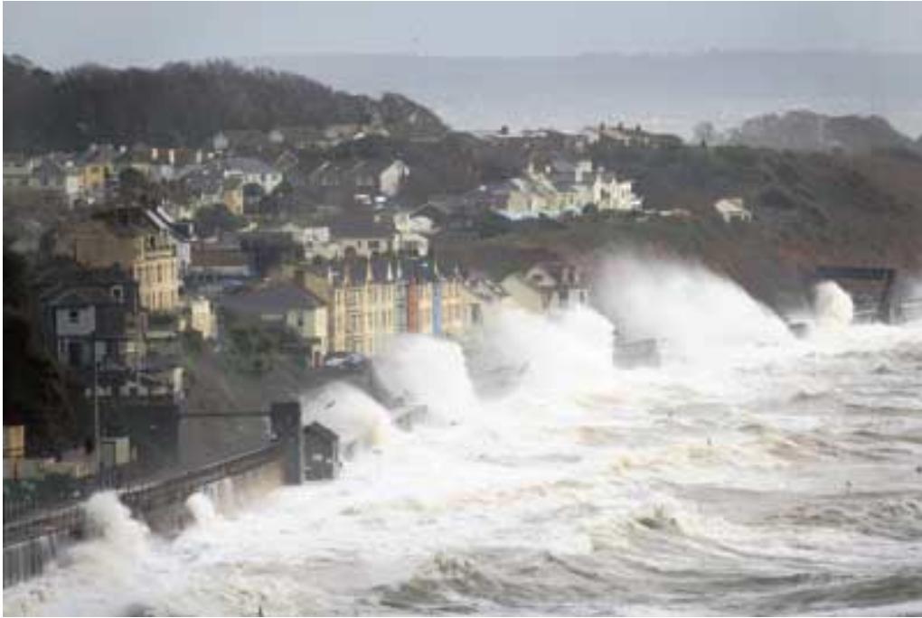
Figure 1.1: A storm hit the Dawlish seawall, (Dawlishnewspapers, 2014)
