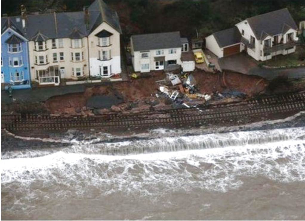
Figure 1.2: Segmental seawall failure at Dawlish, (BBC, 2014)
