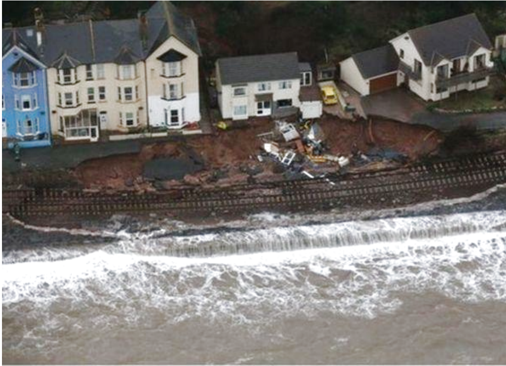
Figure 1.2: Segmental seawall failure at Dawlish, (BBC, 2014)
