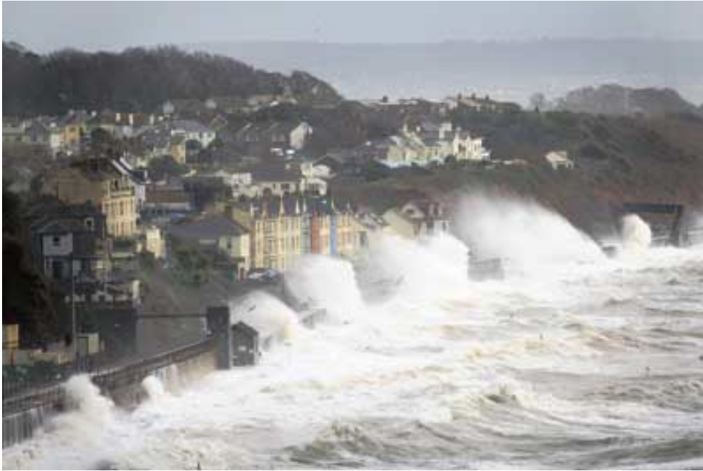
Figure 1.1: A storm hit the Dawlish seawall, (Dawlishnewspapers, 2014)
