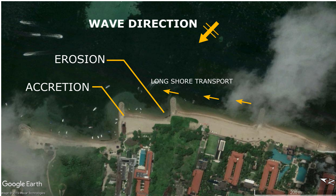
Figure 2.6: Beach protection using groynes, showing the resulting long-shore transport modification at Nusa Dua, Bali (Google Earth)
