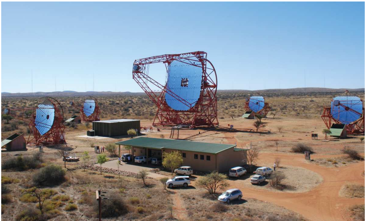
Figure 4.1 – H.E.S.S. site in Namibia with four medium-sized Cherenkov telescopes CT1-CT4, layed in a square configuration from right to left and with one large-sized Cherenkov telescope CT5 in the middle of the array.
