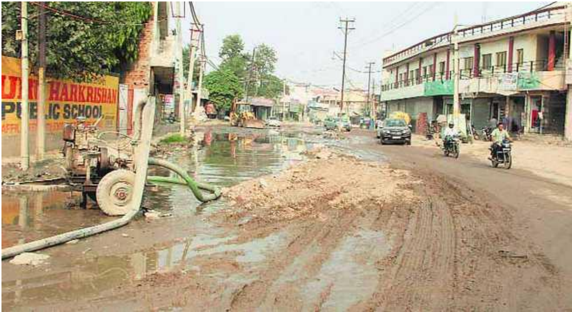
Figure 17: Sewerage work on the
