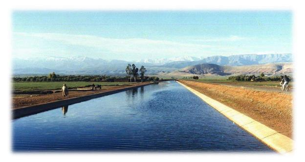
*Figure 4: "Rocade" canal, transporting irrigation water coming from the "Hassan 1" dam located in the neighboring catchment of Oum Erabia.*
