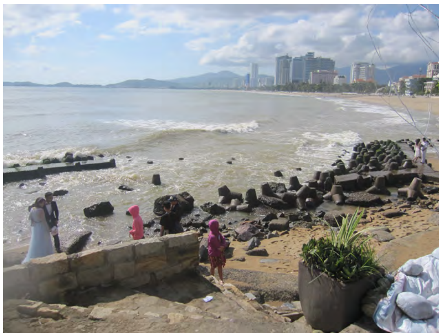
Figure 2.13: Two jetties made from tetrapods at the south of Nha Trang View restaurant. Photo taken at 09h22 06/12/2015.
