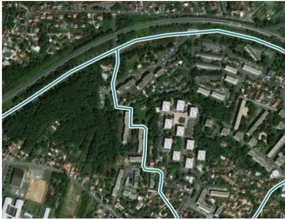
Figure 50 Point A requiring civil works
