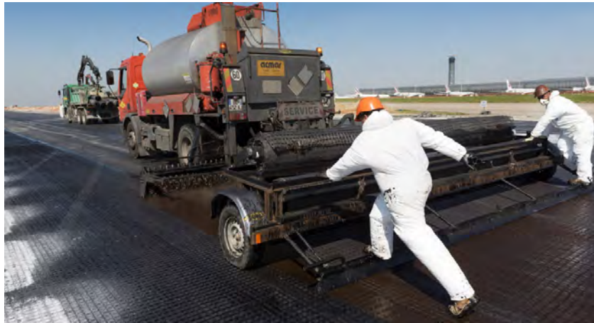
Figure 6.2 – Glass fiber grid installation at Roissy CDG (COLAS)
