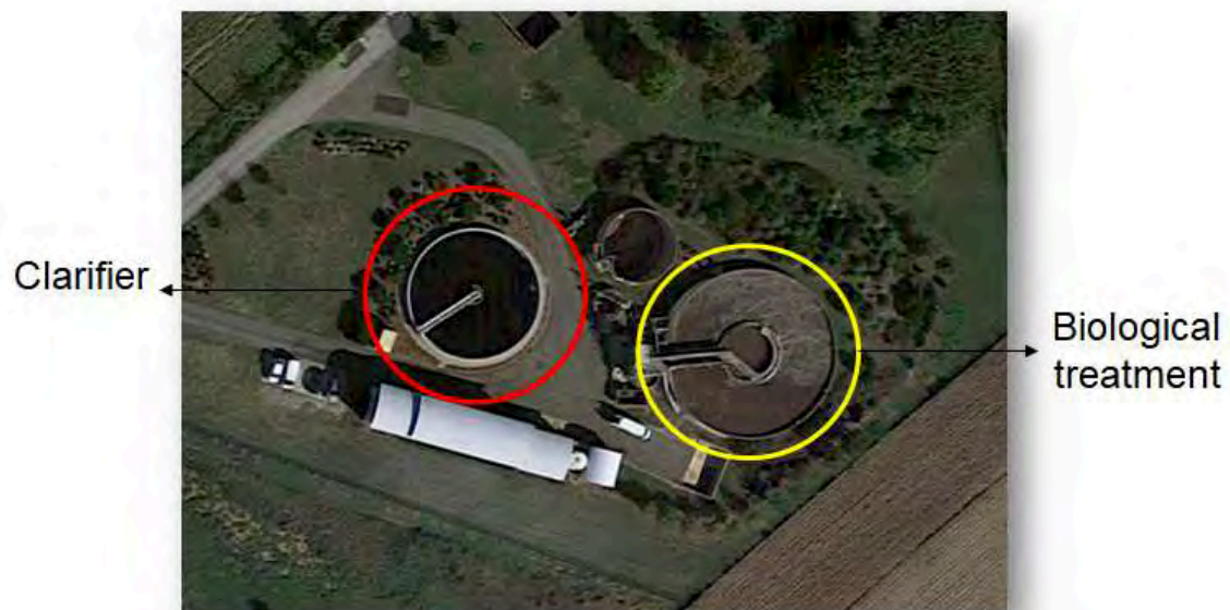
FIGURE 4.2: Aerial view of the Achenheim WRRF
