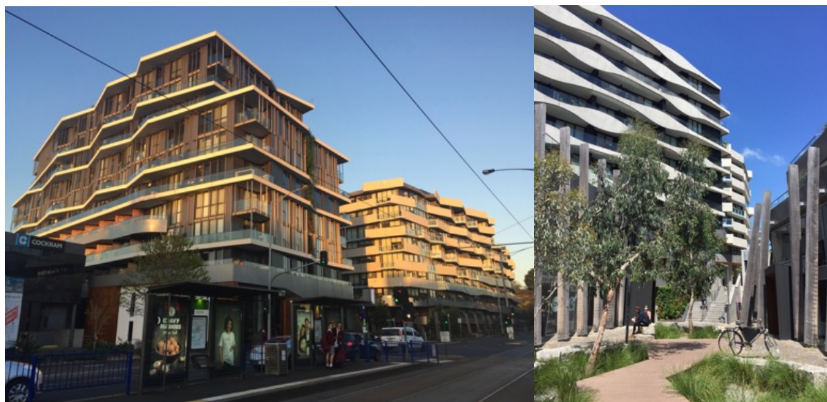
Figure 4.7 and 4.8: The outside façade of Acacia Place from Victoria Street and the internal courtyard leading to the river, November 2018. Photos: L. Dorignon
