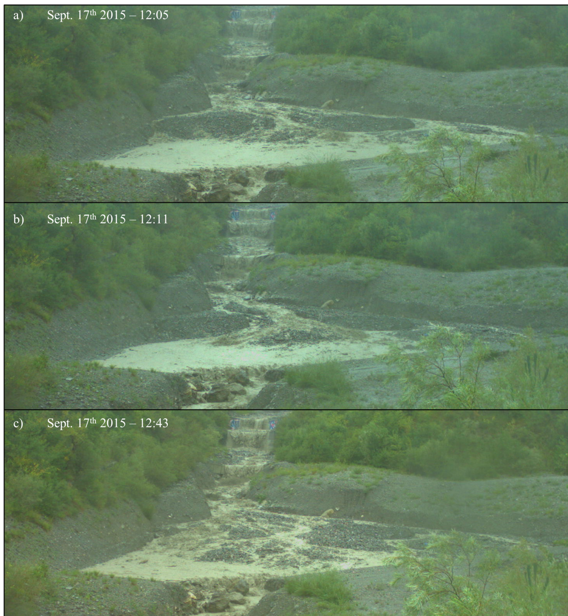
Figure 8.18 – Small debris flood event in the Manival sediment trap on September, 17 th 2015, evidences of cycles of: a) braided channels, b) incision with lobe formation, and c) new braided pattern. Larger events are expected to confirm these encouraging results
