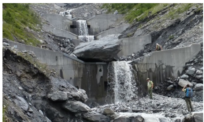
Figure 1.10 – Huge boulder stopped on the check dam series of the St. Antoine torrent upper basin (73 – FRA.) – 2014 (photo courtesy of S. Carladou)
