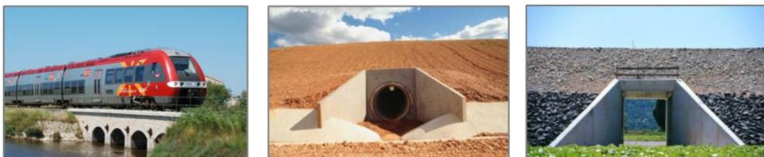
FIGURE I-33: EXEMPLES D'OUVRAGES HYDRAULIQUES DE TRAVERSEE (DE GAUCHE A DROITE: AQUEDUC, BUSE, DALOT)
