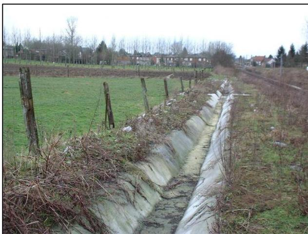
FIGURE I-34: PHOTO D'UN FOSSE REVETU PLACE EN CRETE DE DEBLAI POUR INTERCEPTER LES ECOULEMENTS. L'EAU PLUVIALE EST ENSUITE ACHEMINEE VERS UN EXUTOIRE VIA UNE DECENTE D'EAU OU LA PROCHAINE JONCTION AVEC UN REMBLAI.
