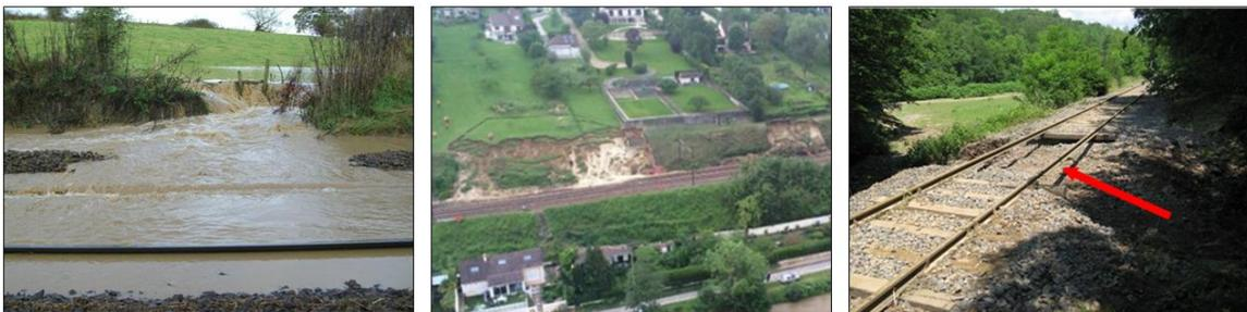
Figure 2: Illustration of surface runoff impacts on railways: from left to right, flood, landslide, and breach in the embankment
