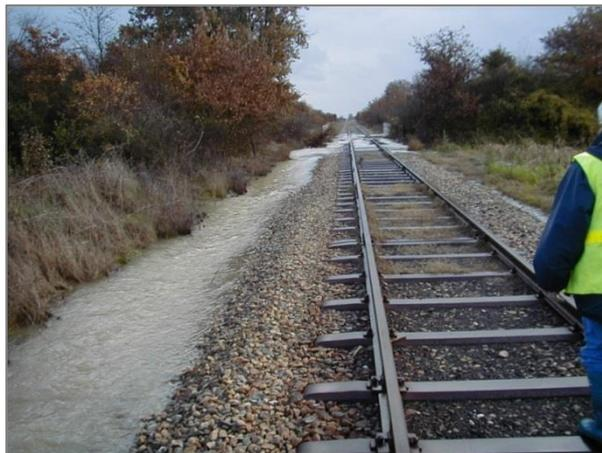
**FIGURE II-38: LE RUISSELLEMENT EST ARRIVE EN UN POINT DE LA VOIE FERREE MAIS A PROVOQUE UN IMPACT ETENDU CAR LA CONFIGURATION DE L'INFRASTRUCTURE A MODIFIE LES ECOULEMENTS.**
