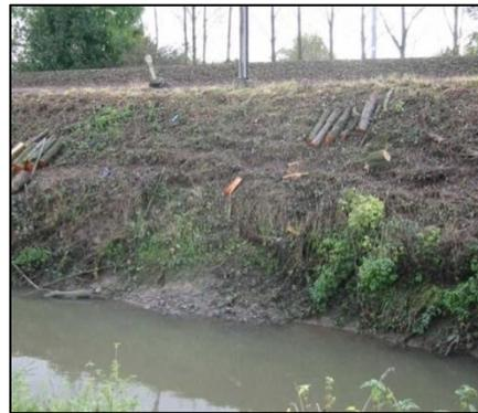
**FIGURE I-52: AFFOUILLEMENT DU PIED DE REMBLAI**
