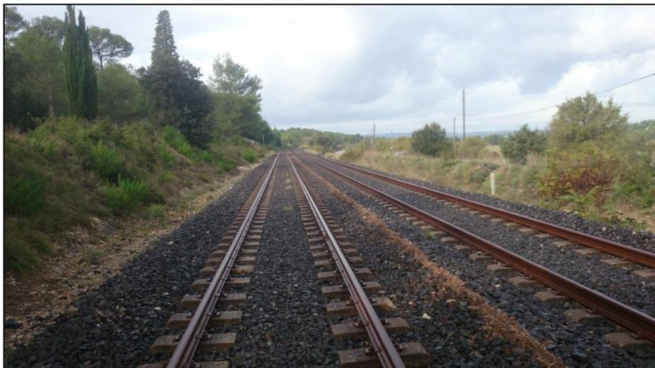
**FIGURE I-57: LES LAISSES DE CRUE ENTRE LES DEUX VOIES NE SERONT PAS FORCEMENT RAPPORTEES PAR LES AGENTS DE TOURNEES PUISQUE NE PRESENTANT PAS DE DANGER DIRECT POUR LES CIRCULATIONS MAIS SONT TEMOINS D'UN PASSAGE D'EAU SUR LA VOIE FERREE ET DONC D'UNE SITUATION DANGEUREUSE A UN CERTAIN MOMENT (DEPARTEMENT HERAULT, 2014).**
