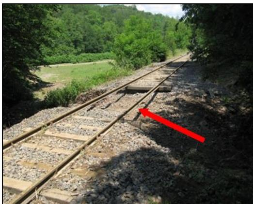
**FIGURE I-50: EMPORTEMENT D'UN REMBLAI FERROVIAIRE**
