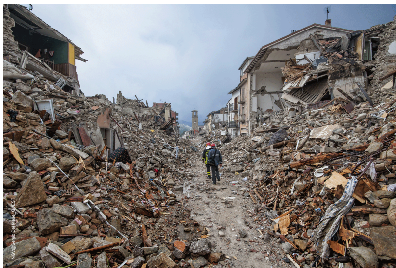
Figure 100 Damage during the August 24, 2016 Amatrice, Italy earthquake (Mag. 6, Int X) (Mesa, 2016; Quest, et al., 2016)
