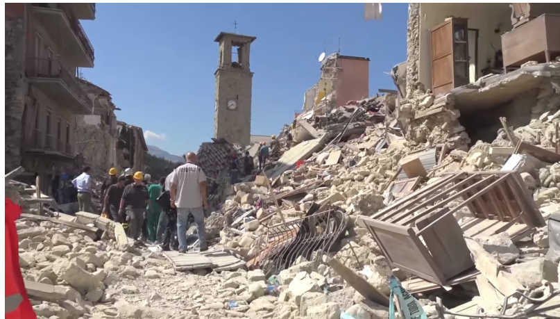
Figure 99 Debris damage during the August 24, 2016 Amatrice, Italy earthquake (Mag. 6, Int X) (Legi il Firenzepost, 2016; Quest, et al., 2016)
