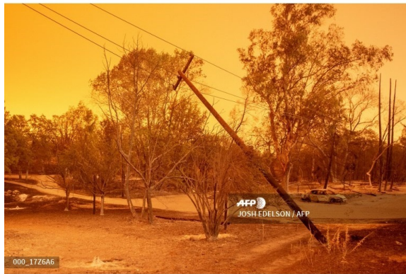
(b) A power pole leans over a burned property during the Carr fire near Redding, California on July 27, 2018 [JOSH EDELSON / AFP #000_17Z6A6].
