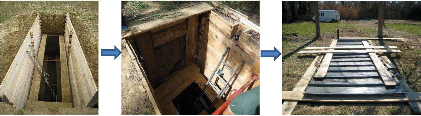
Appendix 3: The big pit covered with a metallic roof
