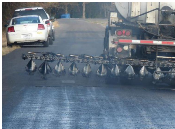
Figure 1.7 - Application of a bituminous emulsion as a tack coat using sprayers
