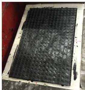
Figure 1.32 - Geogrid placed on a mixture with bituminous emulsion sprayed on it
