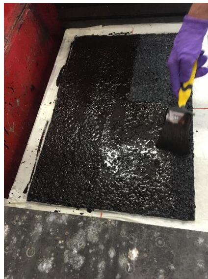
Figure 3.2 - Tack coat application on the lower layer of bituminous mixture using a brush
