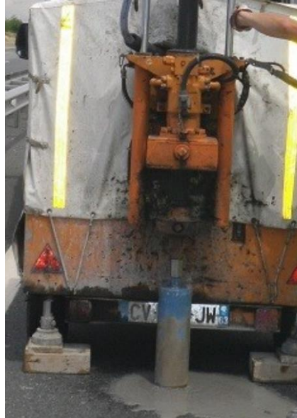
Figure 1.13 - Core drilling machine in use
