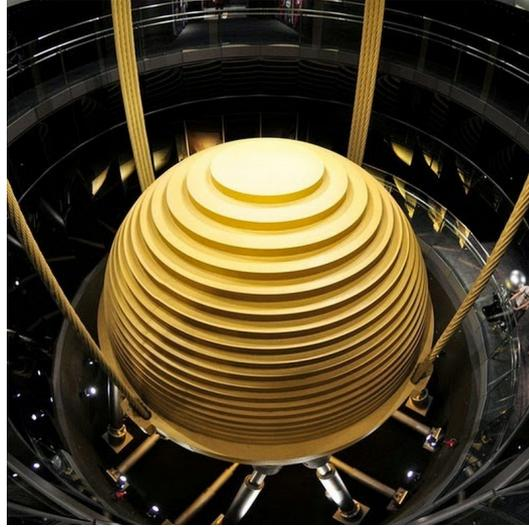
Figure 0.3 – Tuned mass damper used in the *Taipei 101* skyscraper.
